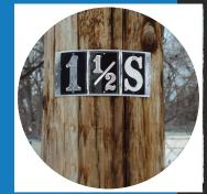
The BDX is a bevel-edged plaque (0.016" aluminum) with 2-½" tall characters de-bossed into a 3-¼" x 2-¾" rectangle. Each figure has two .10" mounting holes, top and bottom. Mounting frames for grouped characters are available in sizes holding 2 to 8 characters, in either horizontal or vertical orientation. Frames are made of .020" aluminum with mounting holes at each end.
